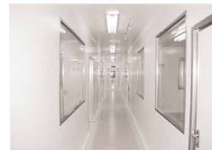
Class 100 Clean Room
